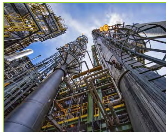
Petra Nova in Texas (USA) is the world's largest post-combustion carbon capture system, capturing CO 2 produced by burning coal for use in enhanced oil recovery (EOR).
