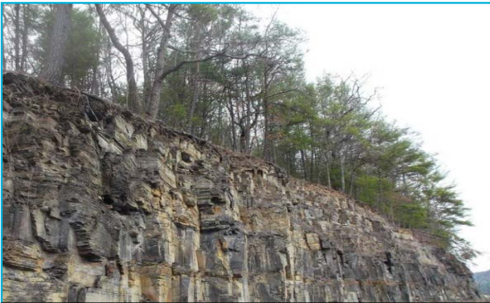
Parallel, vertical, orthogonal natural fracture faces (joint sets) in an outcrop of organic-rich Millboro Shale (Marcellus equivalent), Clover Creek, VA. Photo by Dan Soeder, 2014.
