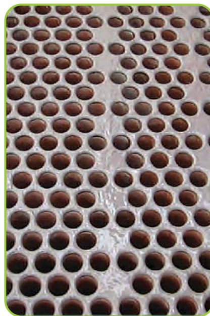
Examples of Cleaned and Fouled Condenser Surfaces
