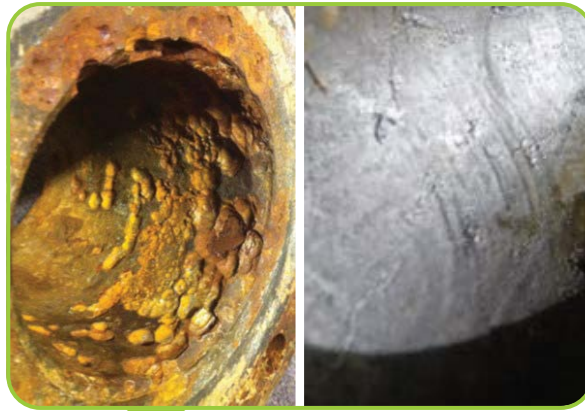
Typical Mic Damage to Spool (Left) vs. Dragx™ Treated Spool After Six Months (Right)
