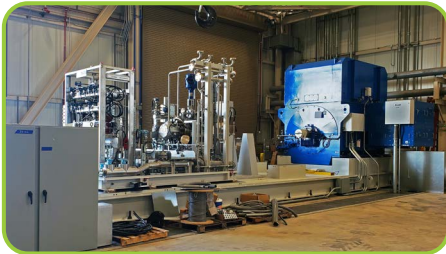
Turbine Skid and Bypass Compressor
