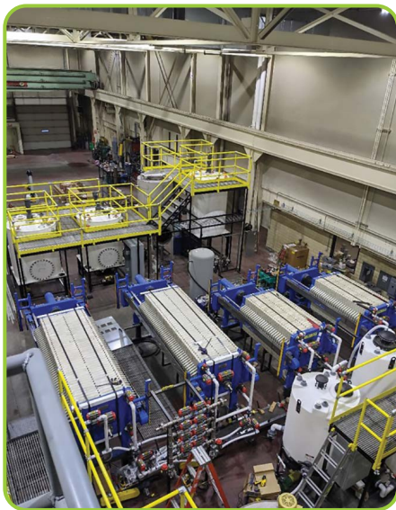
UND Coal and Mineral-Rich Tailings Filter Presses, with the Liquid Processing Tanks Featured in the Background
