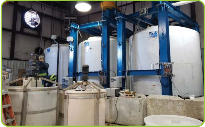
Sulfuric Acid Bioreactors
