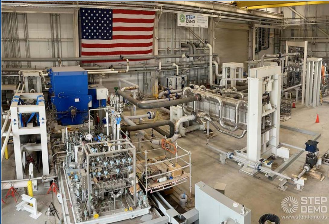
Supercritical Transformation Electric Power 10 MWe pilot plant.
