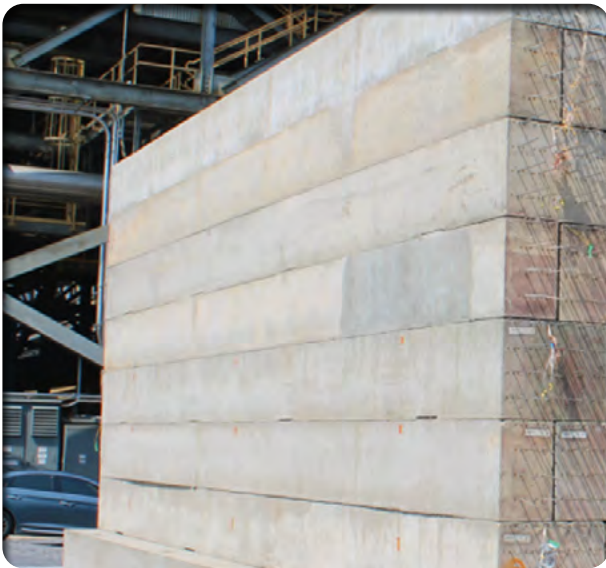
Finalized, assembled CTES stack at Plant Gaston.
