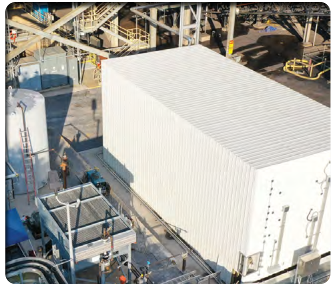
Finalized, assembled CTES stack at Plant Gaston.
