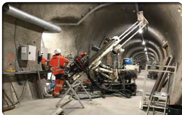
Drilling and coring at Mont Terri with 52mm ID casing.
