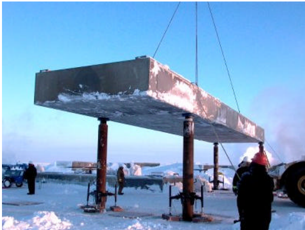
Figure A-3. Setting the First Platform Module
