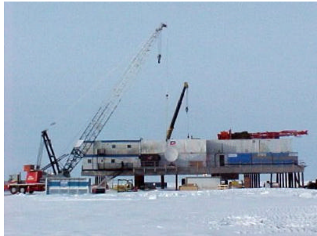
Figure A-4. Assembling the Platform
