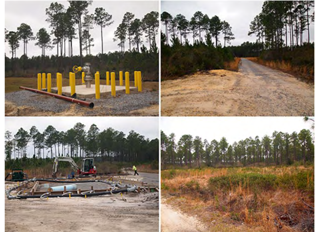
Photographs of existing Gulf Power wellfield. Photos clockwise from upper left: Eocene Injection well EIW-4; gravelled access road; pump station under construction; cleared and permitted drilling pad location for future well
