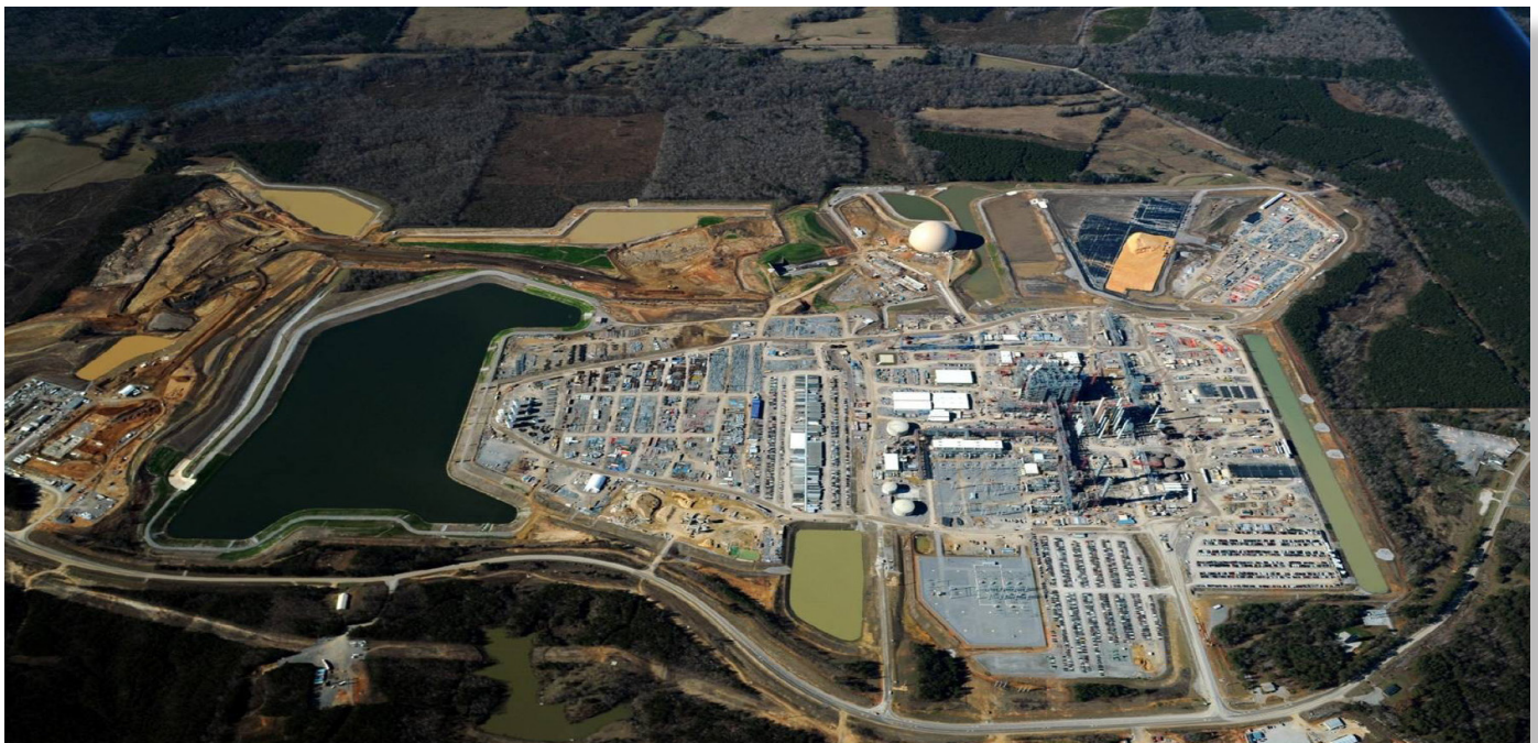
Aerial View of Kemper County Energy Facility (December 2012)
