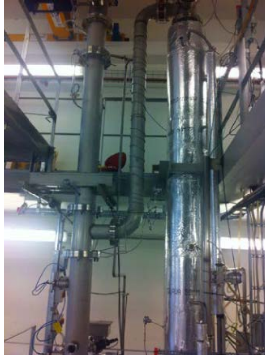
Additional Water Wash column
