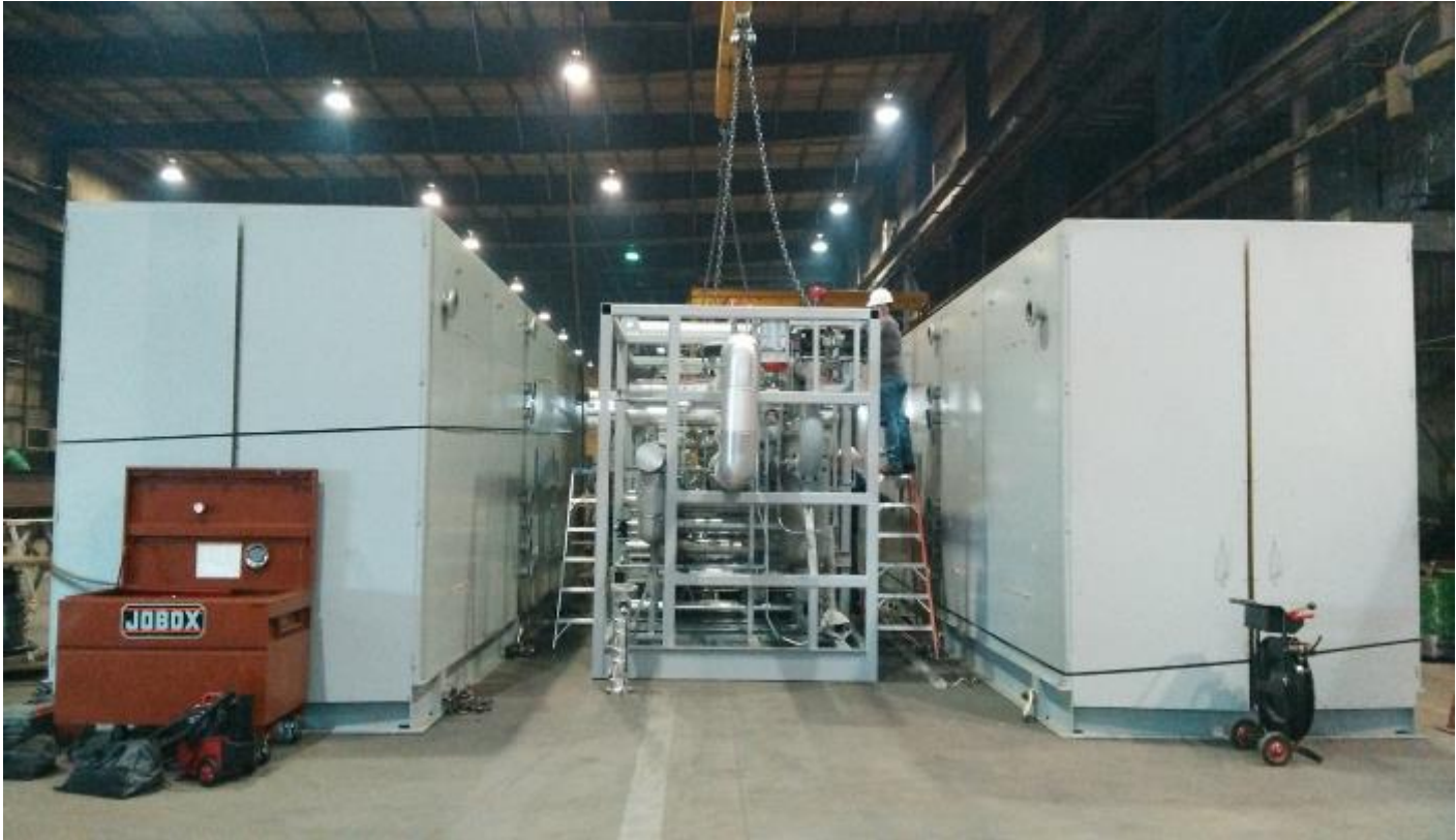
Skids set in place at Fabrication shop for FAT testing
