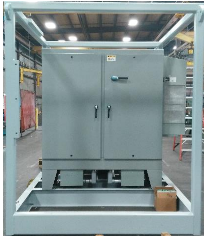
High Voltage Power Enclosure
