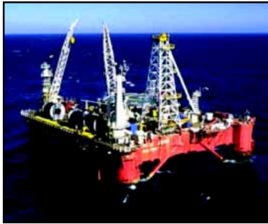
Caldive, Inc.'s Uncle John semi-submersible drilling vessel
