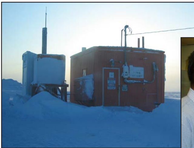
Figure 3. Well housing and methanol tank (methanol injection is used to mitigate hydrate formation in the production string) at the East Barrow No. 14 well.
