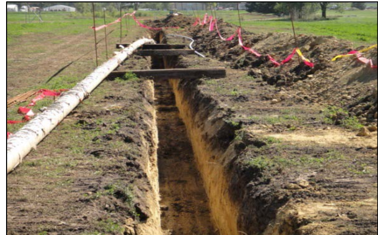
8" High Pressure transmission Line
