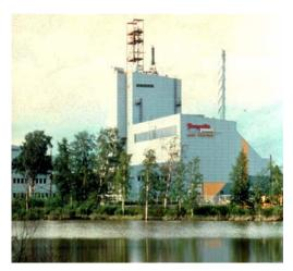
26 test runs. The tested fuels include coal (Polish, Colombian, coke, German lignite) and biomass (wood, paper mill wood waste, forest residue, willow, straw, alfalfa) and mixtures of coal and biomass. Gas generated in the plant is combusted in a heat recovery boiler producing district heat for the city of Tampere.
