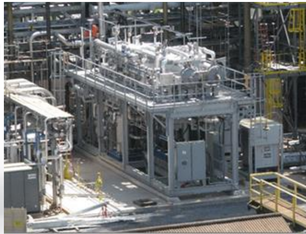
Existing MTR Membrane Module (20 TPD evaluated at NCCC)
