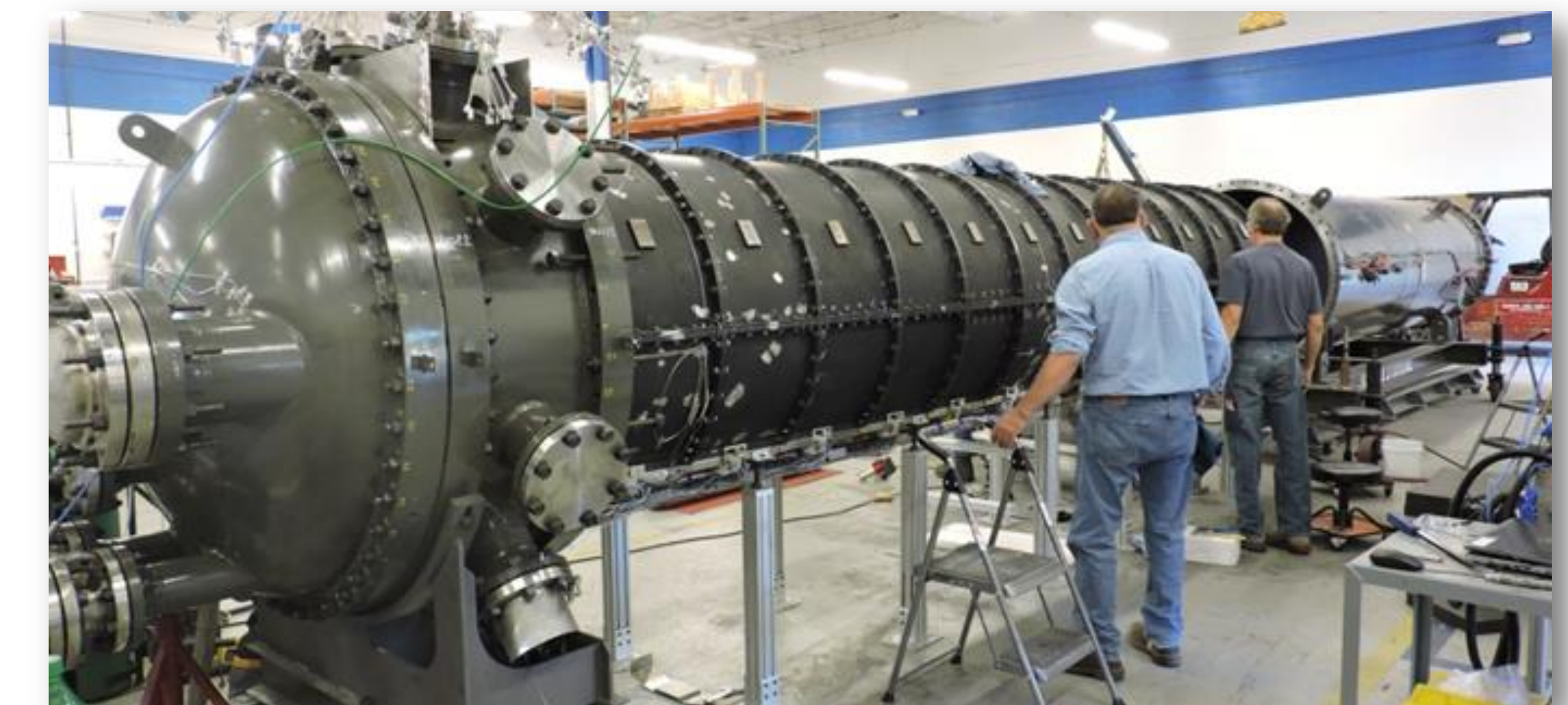
Fuel Cell Vessel Assembly
