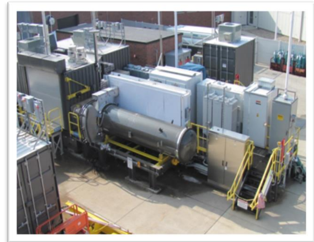
200 KW Fuel Cell Vessel
