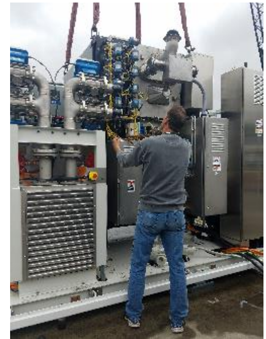
100 kW Stack Module Integration
