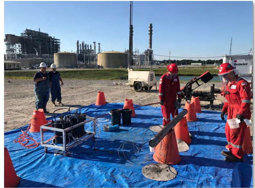
MPC 10-4 Epoxy injection for core preservation
