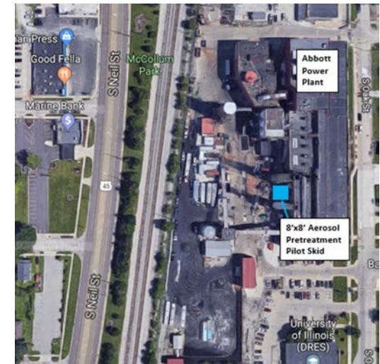
Abbott plant aerial view
