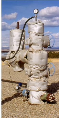
*Insulated CO<sub>2</sub> source wellhead*
