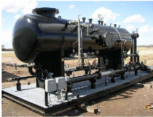
*Separator for separating produced fluids (oil, water, and gas)*
