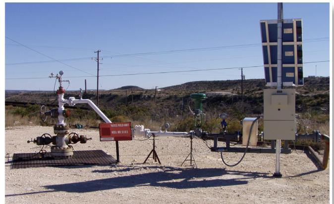
CO<sub>2</sub> injection wellhead
