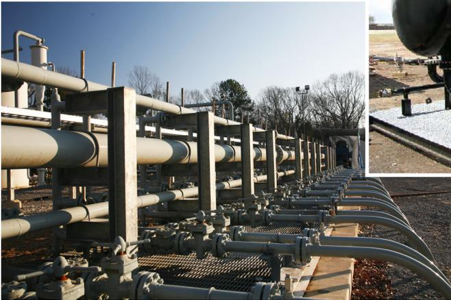
*Well production manifold to allow individual testing of wells*
