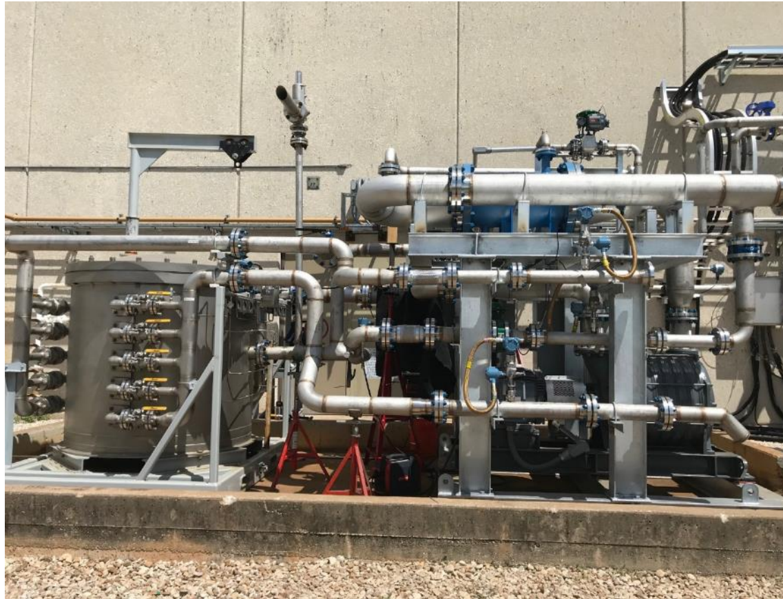
MTR's Plate-and-Frame Membrane Skid
