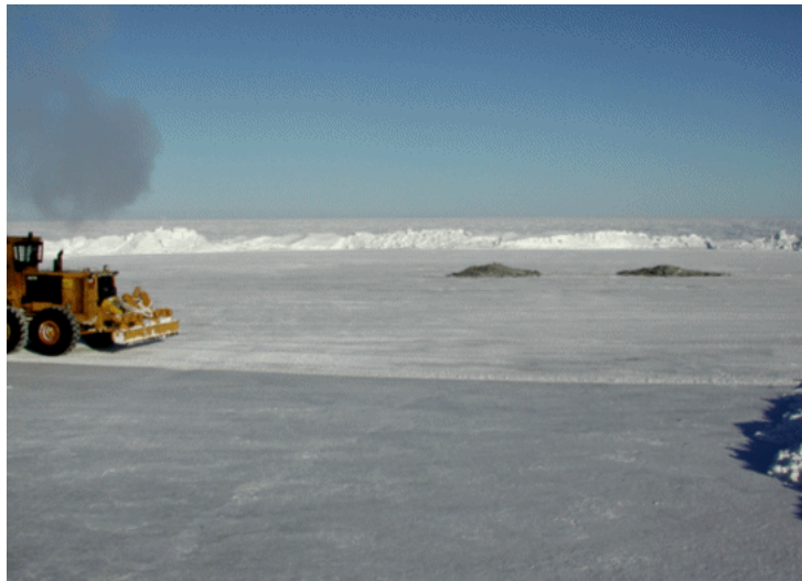
Figure 4. Final Stage of Platform Removal and Site Remediation
