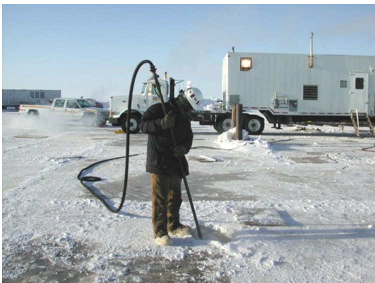
Figure 21. Vacuuming Platform Leg Holes after Leg Removal
