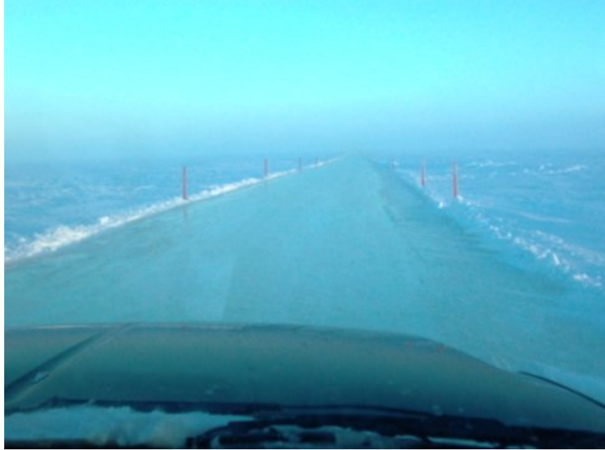
Figure 7. Ice Road after Maintenance Run
