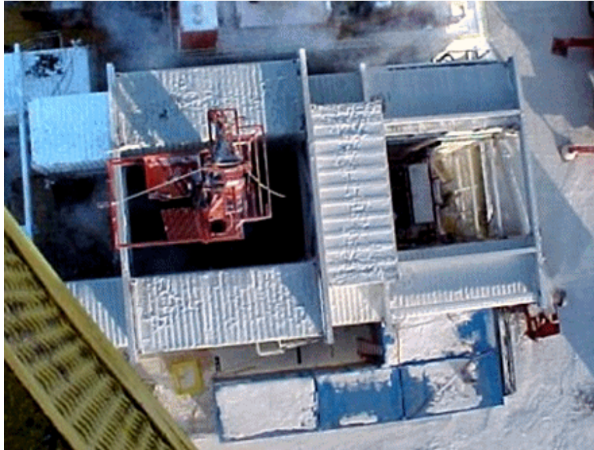
Figure 2. Overhead View of Coring Rig (red rig mast was covered during operations) and Mobile Core Laboratory (four blue modules at bottom)
