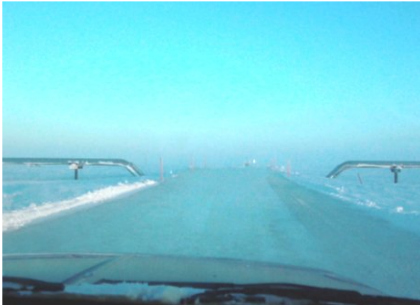
Figure 8. Pipeline Crossing on Ice Road
