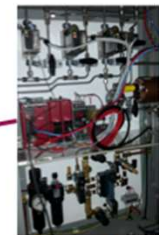
3-channel gas dosing system
