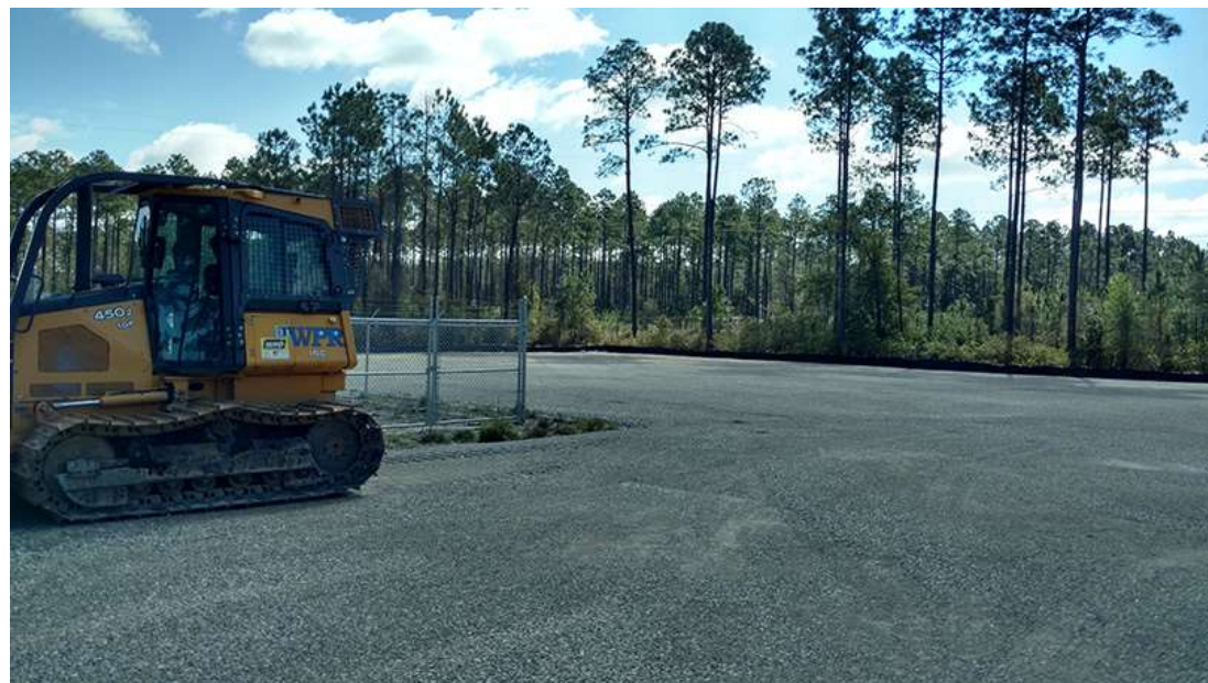
Newly constructed drill pad at Plant Smith for injection well TIW-2
