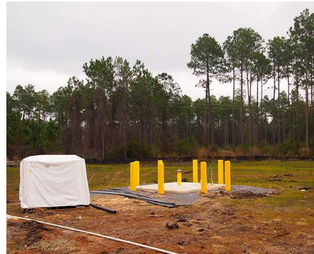
Permanent monitor well installed within 150 ft of injection well is sampled quarterly for water quality impacts associated with injection
