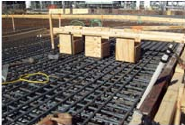
Installation of guy wire anchor points
