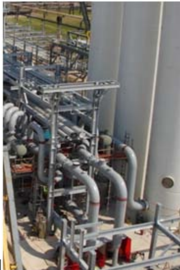
CO 2 Surge Tank Piping and Silencers/ Exchangers
