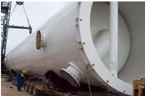
Preparing to set CO 2 Surge Tank
