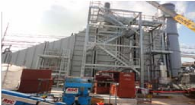
CO 2 Surge Tank Piping and Silencers/ Exchangers
