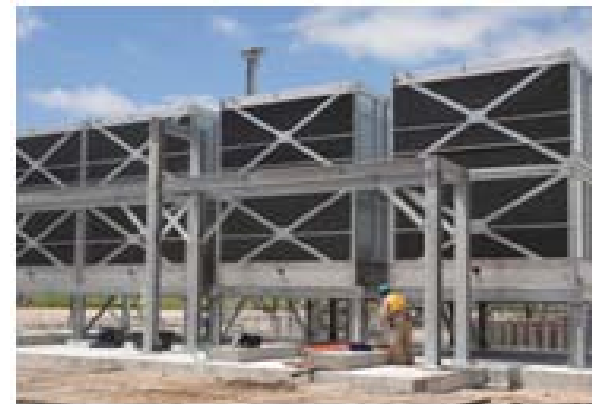
Erection of Cooling Tower
