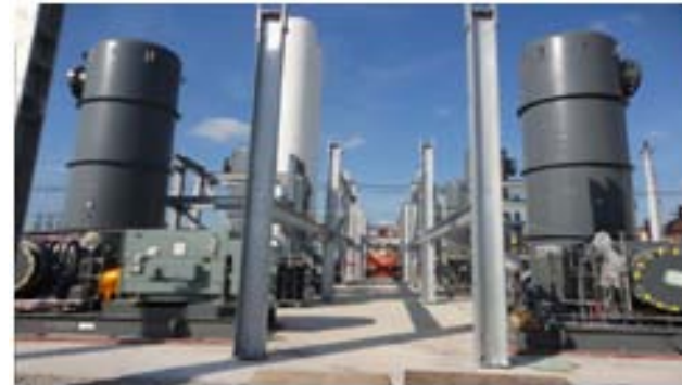
VSA Unit and Piping Support
