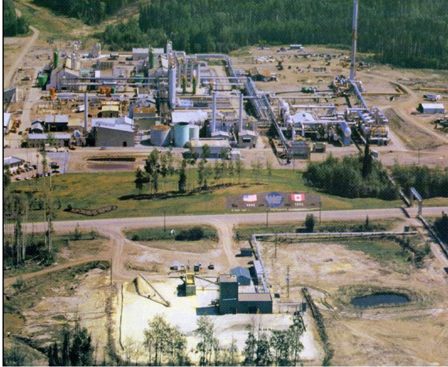
Figure 2. Fort Nelson gas plant, British Columbia, Canada.
