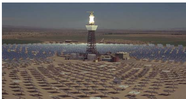
Solar Power Tower
