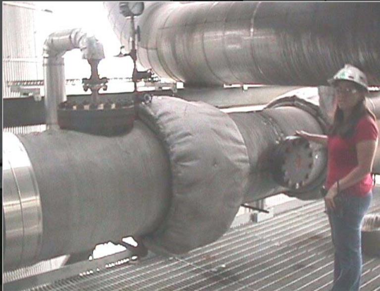
We have also installed an additional venturi scrubber upstream of the COS hydrolysis KO drum. This provides protection for the COS hydrolysis superheater and catalyst bed from particulate fouling in case the upstream syngas scrubbers malfunction.
