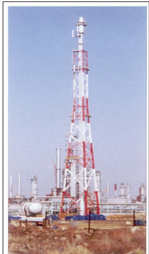
Figure 2.1-9. Typical Flare Derrick with a Single Flare
