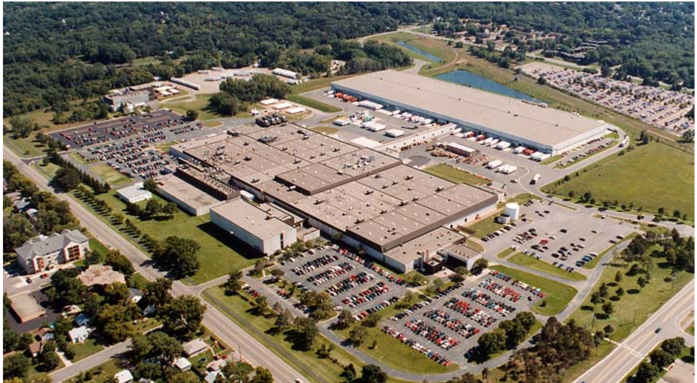
Cummins Power Generation Americas Minneapolis Headquarters and Manufacturing
