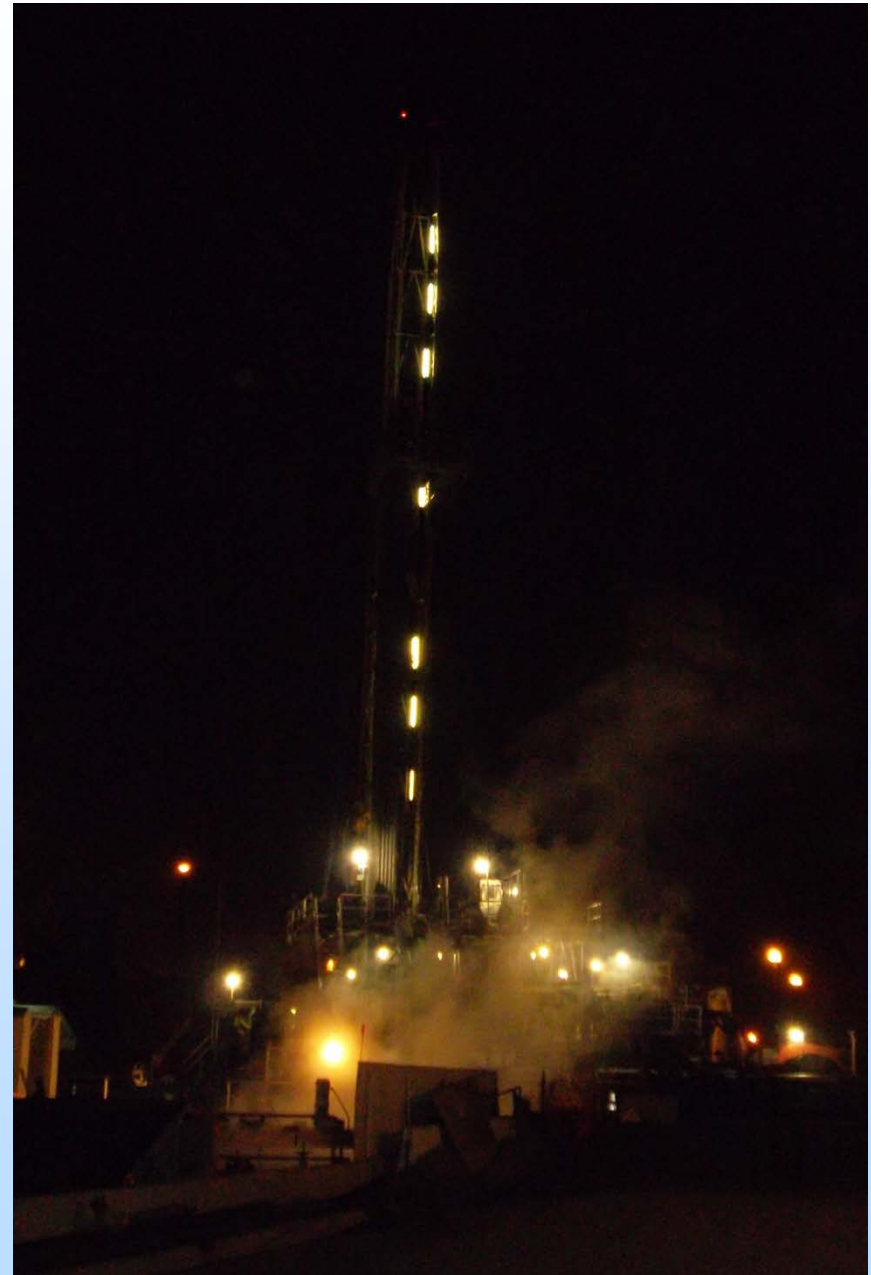
DOE# 2 well completed Mar 18, 2014
