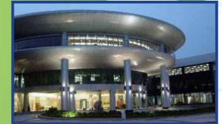
China Technology Center Shanghai, China
