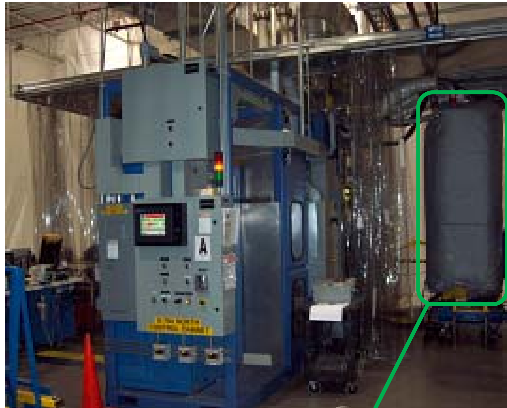
100 kW PAFC test stand with CSA in background
