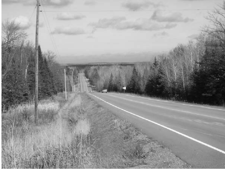
Figure 3.2-4. View of CR 7 Near West Range Site Looking North
