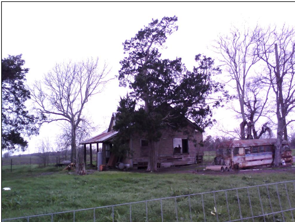
Figure 5.15 Historic standing structure HSS-FB-5 looking northeast
