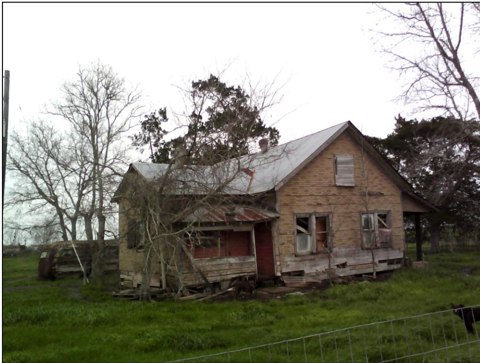
Figure 5.14 Historic standing structure HSS-FB-5 looking south
