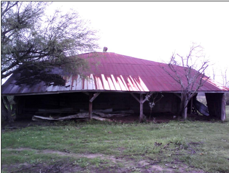
Figure 5.7 Historic standing structure HSS-FB-2 looking northeast
