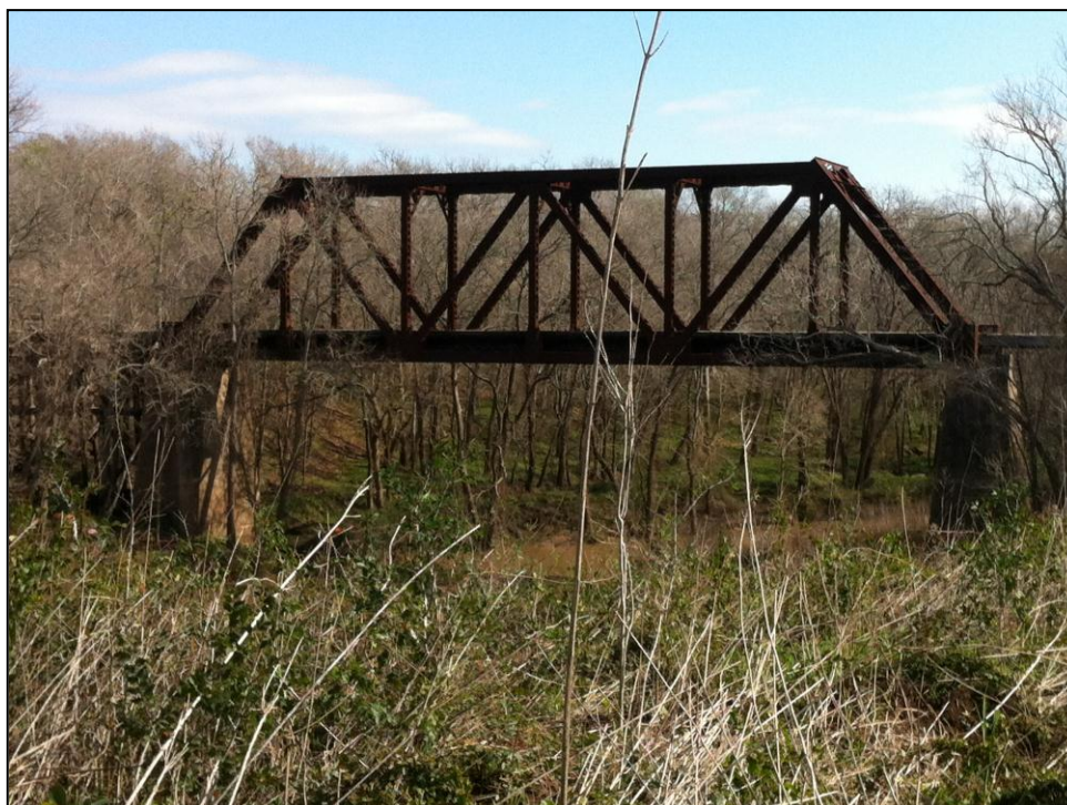
Figure 5.16 Historic standing structure HSS-FB-6 looking north
