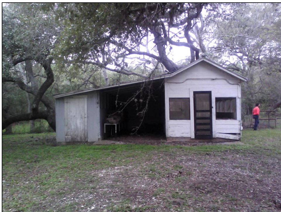
Figure 5.52 Historic standing structure HSS-JK-1 looking northeast
