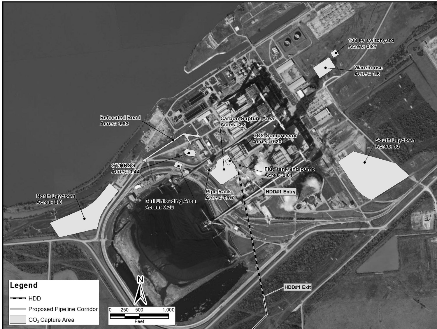
Figure S-3. Aerial Photo of W.A. Parish Plant Showing Areas Related to CO 2 Capture Facility Construction and Operations
