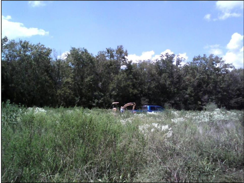
Figure 18: San Bernard River – East HDD, Pre-Excavation (top) and Post-Excavation (bottom) Photographs
