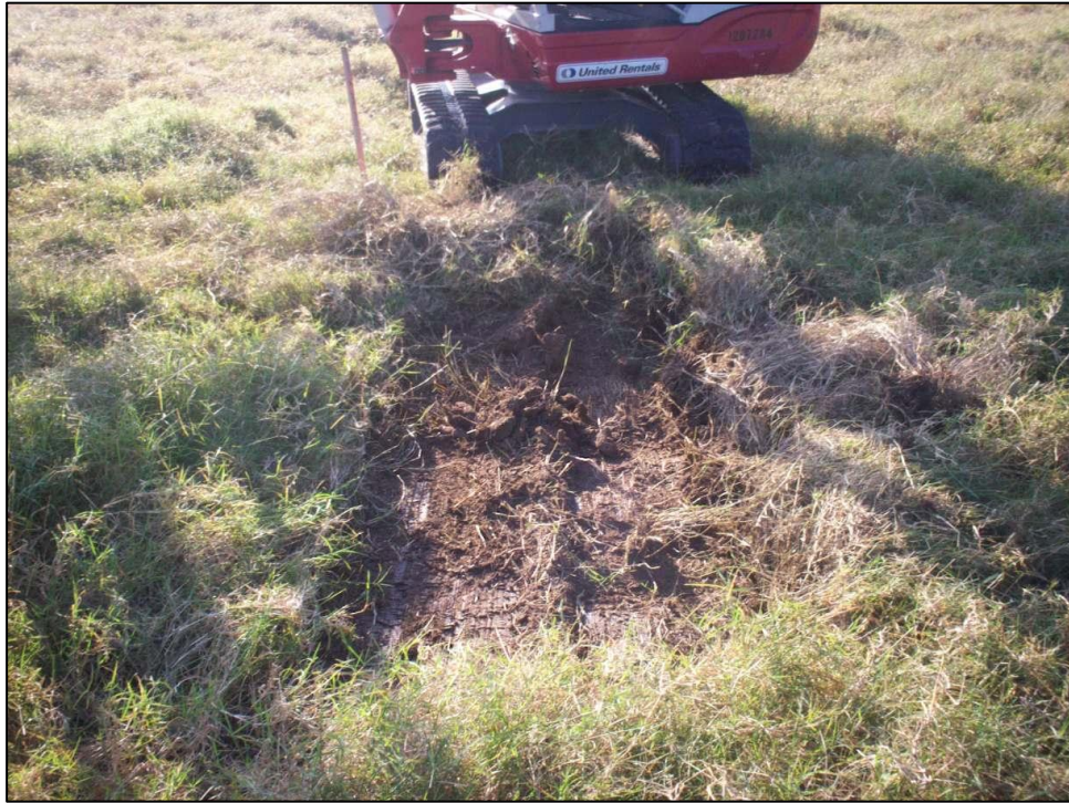
Figure 22: Colorado River – East HDD, Pre-Excavation (top) and Post-Excavation (bottom) Photographs
