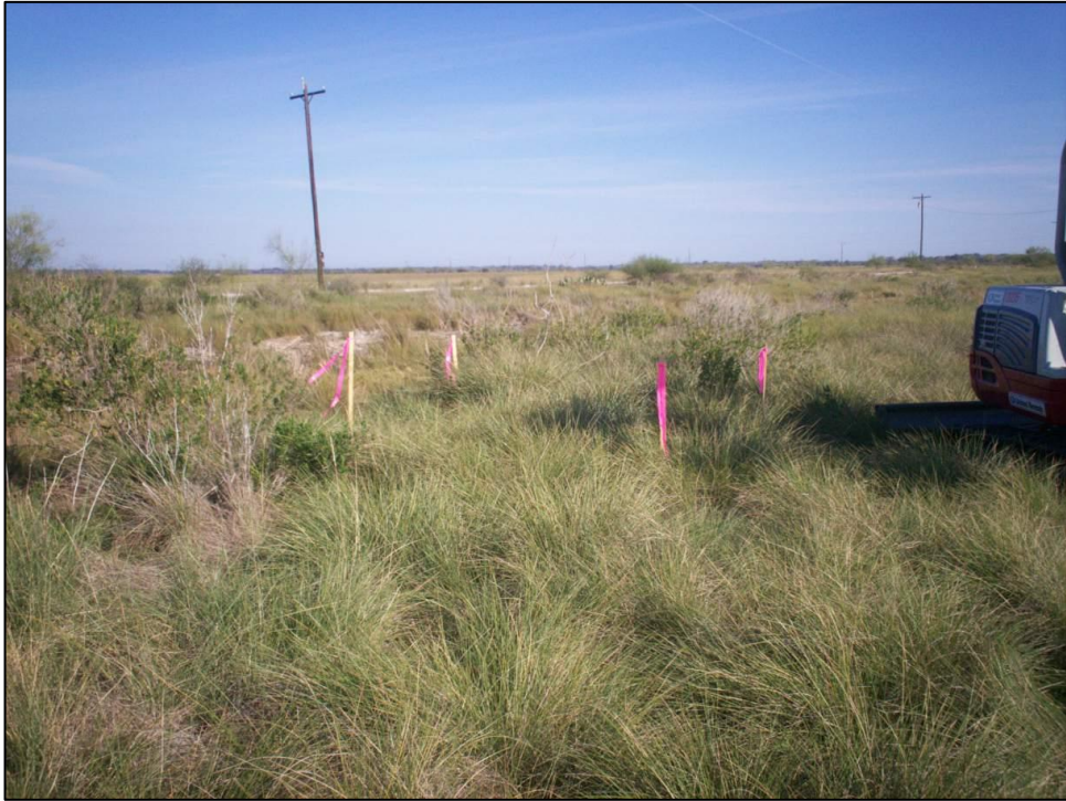
Figure 28: Menefee Bayou – East HDD, Pre-Excavation (top) and Post-Excavation (bottom) Photographs
