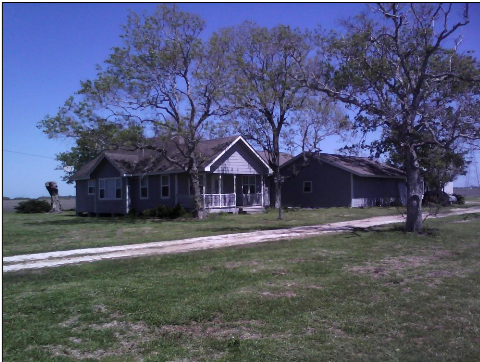
Figure 5.36 Historic standing structure HSS-WH-4 looking northeast
