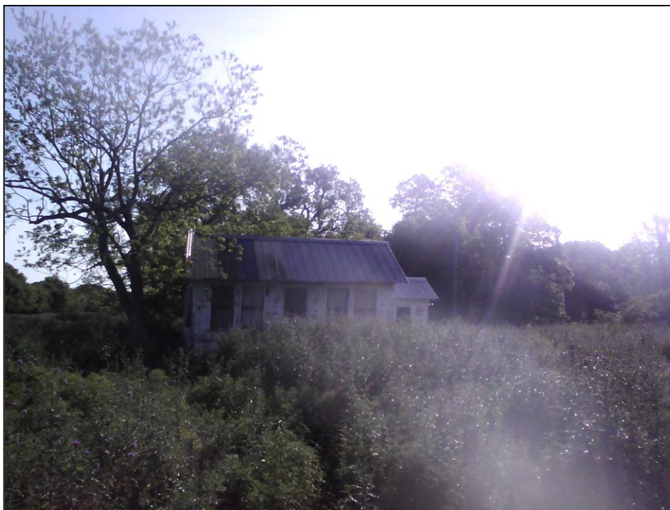
Figure 5.22 Historic standing structure HSS-WH-1 looking east
