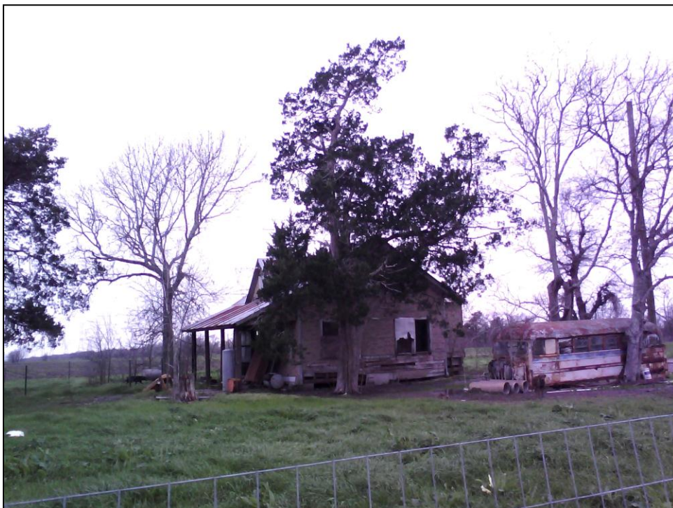
Figure 5.15 Historic standing structure HSS-FB-5 looking northeast
