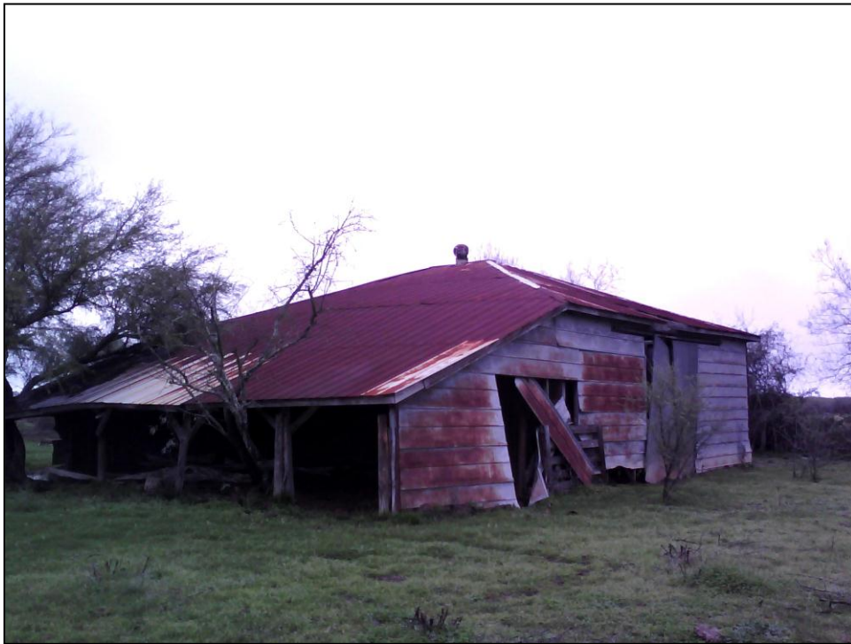
Figure 5.6 Historic standing structure HSS-FB-2 looking east
