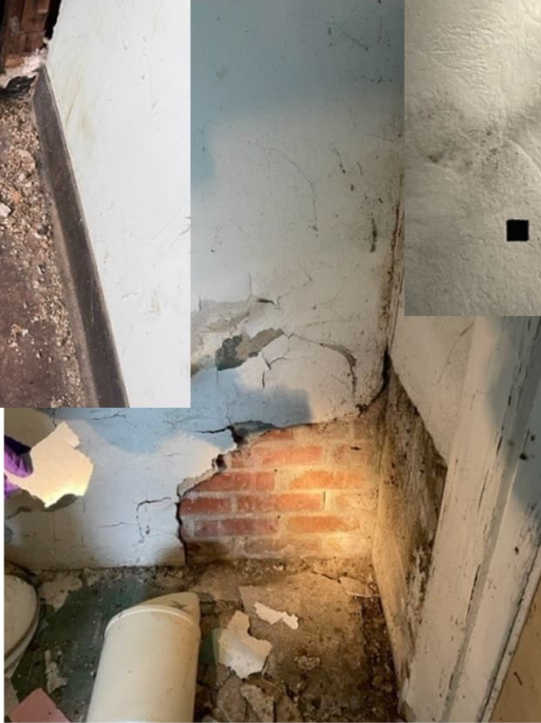
Examples of significant water damage and decay
