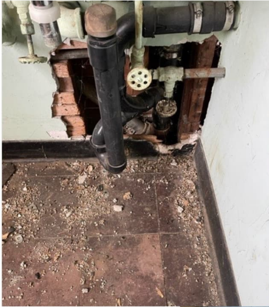
Examples of significant water damage and decay
