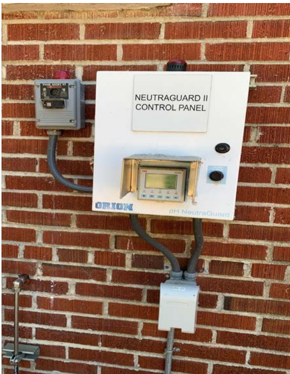
Photos 3.2.6.2a and 3.2.6.2b: Elementary Neutralization System.
