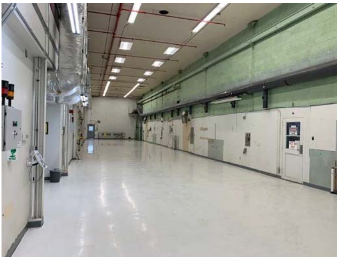
Photo 3.2.2.2: B-28 Fire Damage Rebuild
