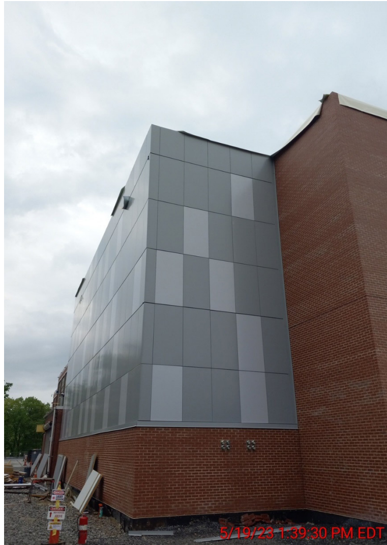
Photo 3.3.2.1: B-83 CDAML – Building Addition.
