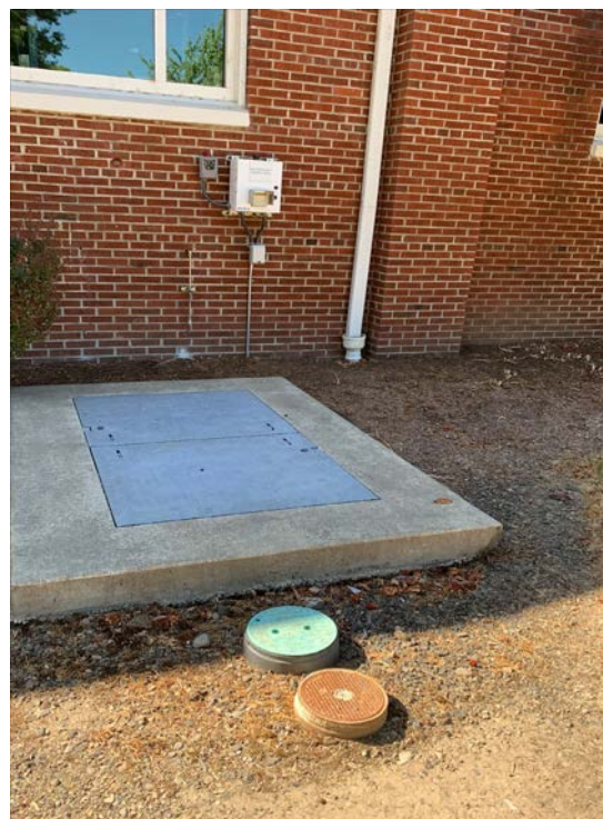
Photos 3.2.6.2a and 3.2.6.2b: Elementary Neutralization System.
