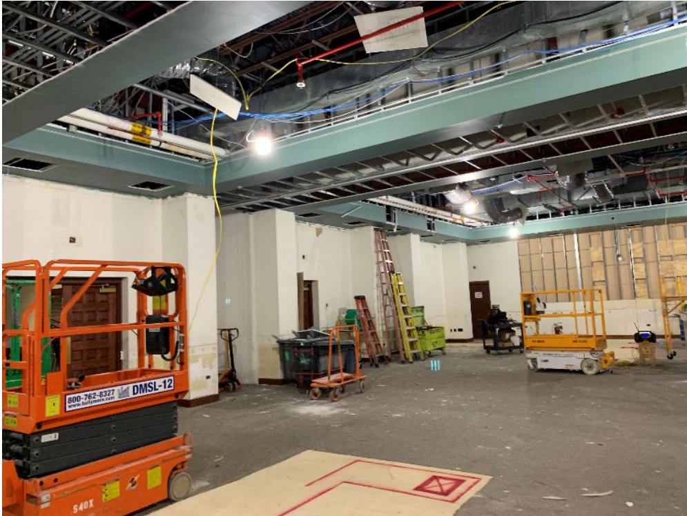
Photo 3.3.2.2: B-922 Conference Center Renovation – Room 106.
