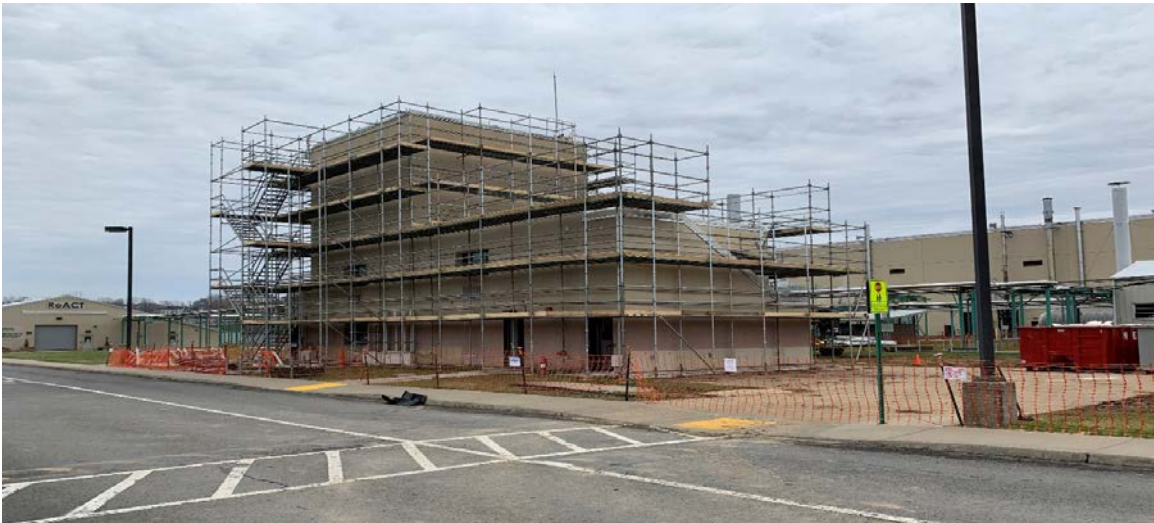
Photo 3.5.2.3a: B-7 Previous Security Building Demolition in Process.
