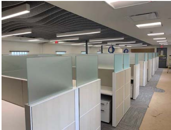
Photo 3.2.2.3: B-17 East Wing Renovation.
