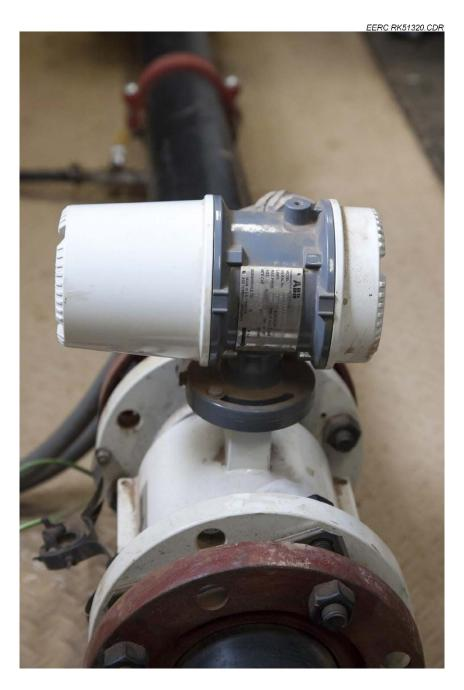
Figure D-42. Image of FEP 300 ABB electromagnetic flowmeter in field.
