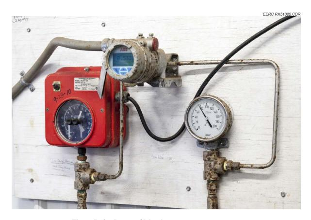
Figure D-36. Image of Murphy pressure gauge sensor.
