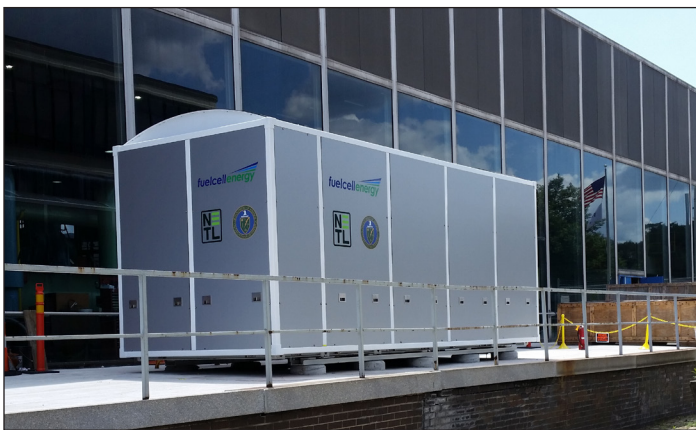
FIGURE 2. FuelCell Energy 200 kWe Prototype System. Photo courtesy of FuelCell Energy
