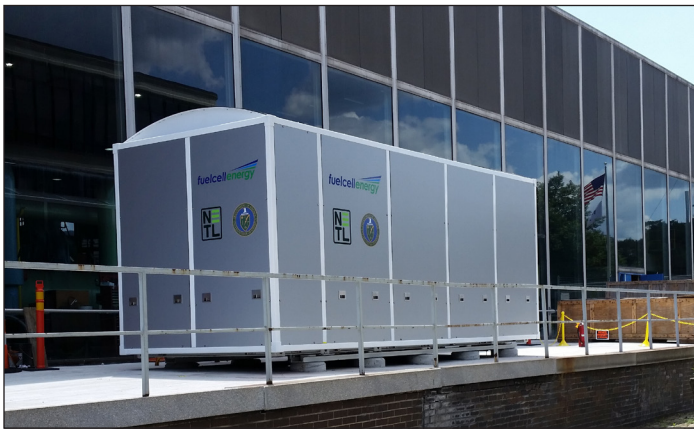
FIGURE 2. FuelCell Energy 200 kW Prototype System. Photo courtesy of FuelCell Energy
