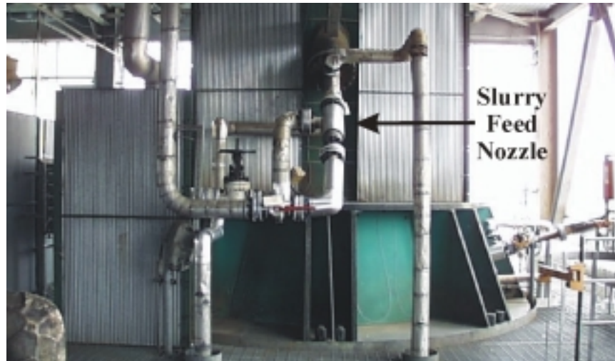
Figure 5.3.2B: Second Stage Gasifier Slurry Feed Nozzle
