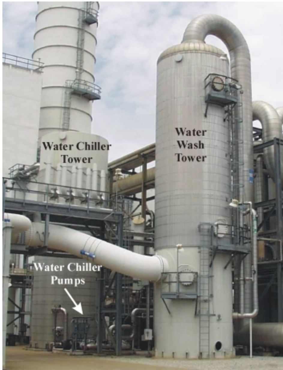
Figure 5.1.2A: Water Wash System
