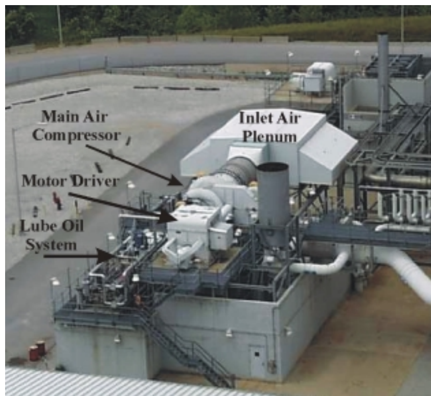
Figure 5.1.1A: Main Air Compressor
