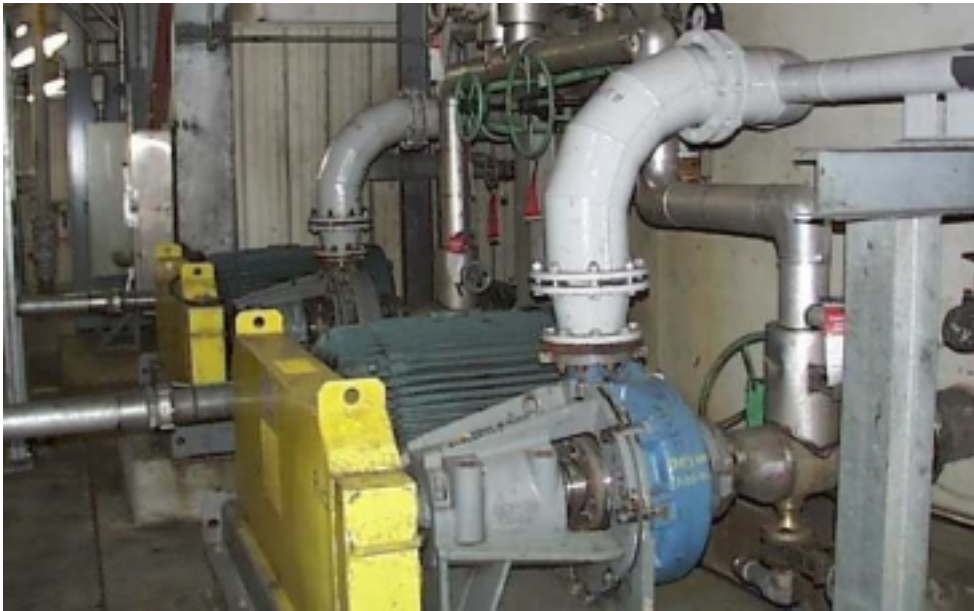
Figure 5.2.3B: Slurry Recirculation Pumps
