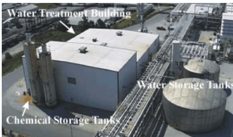
Figure 5.4.3A: Water Treatment/Handling System
