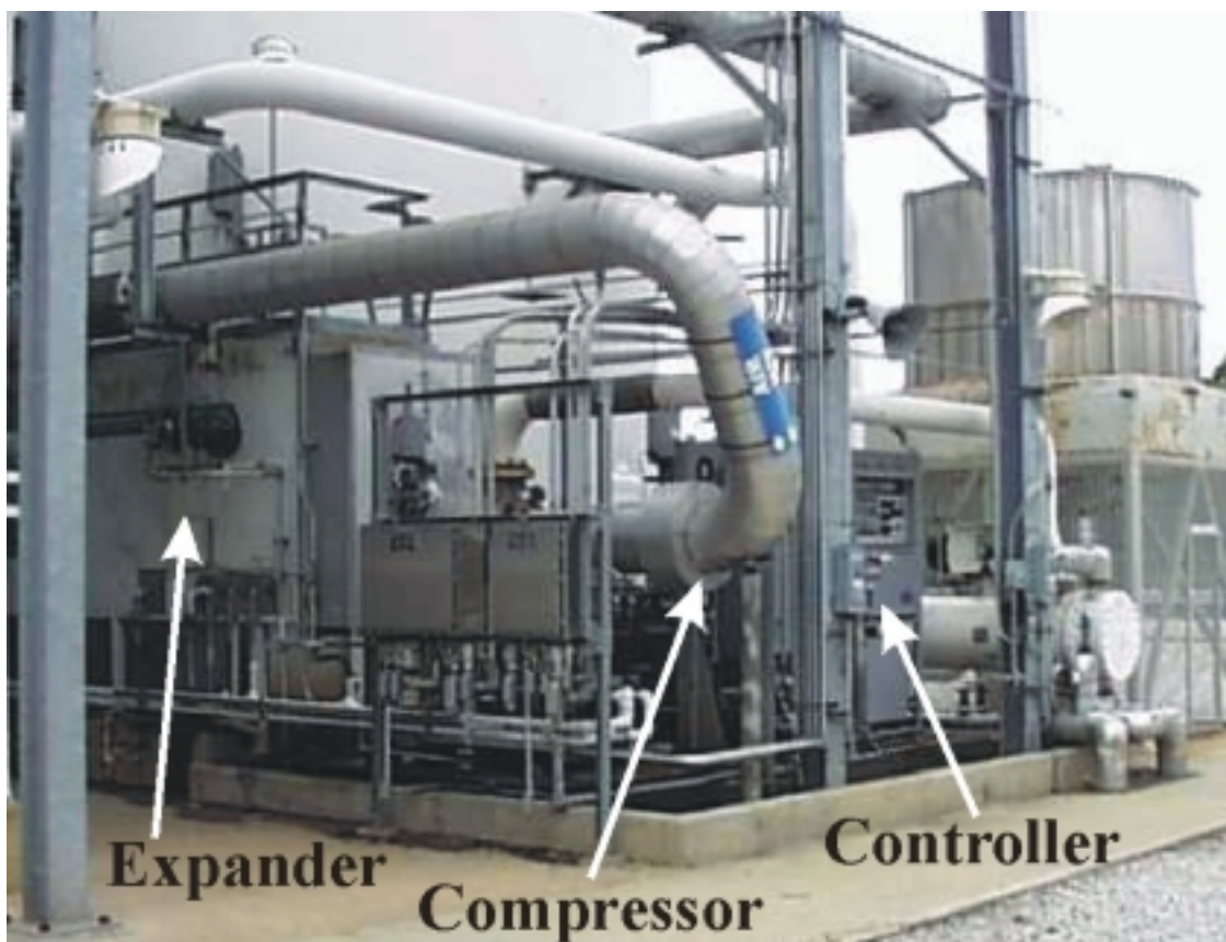
Figure 5.1.4B: Compressor/Expander Skid
