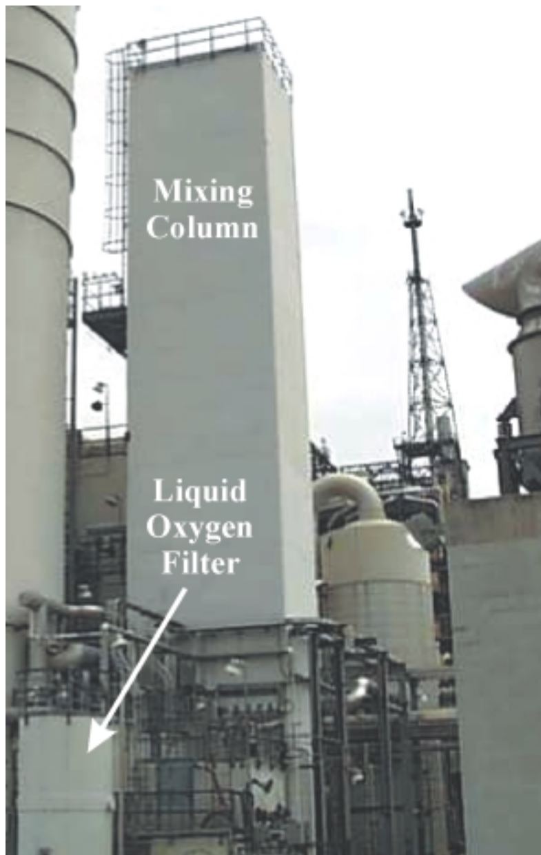
Figure 5.1.6A: Equipment Associated with Oxygen Mixing System
