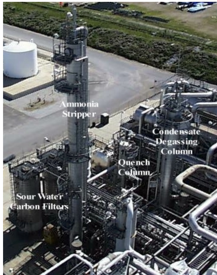
Figure 5.3.13A: Sour Water Treatment System Major Equipment
