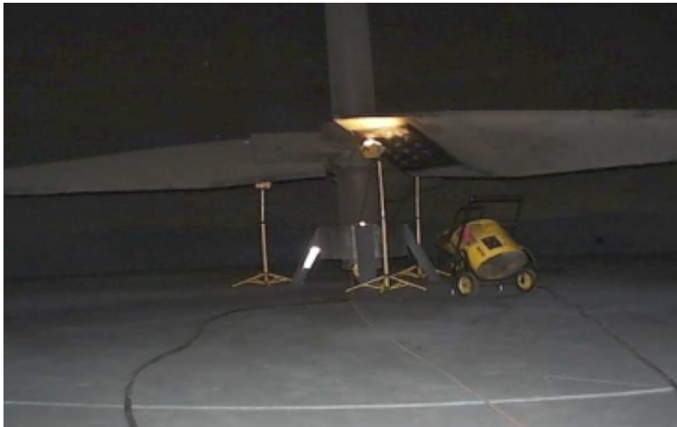
Figure 5.2.3A: Slurry Storage Tank Agitator
