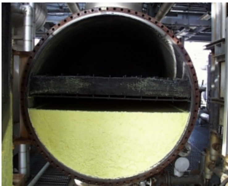
Figure 5.3.12B: Sulfur in No. 4 Sulfur Condenser as a Result of a Plugged Seal Leg
