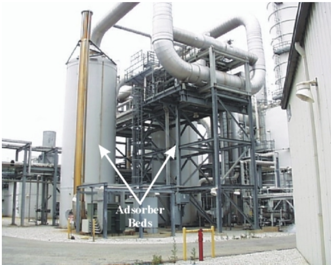
Figure 5.1.3A: Adsorber Beds for the Air Purification System
