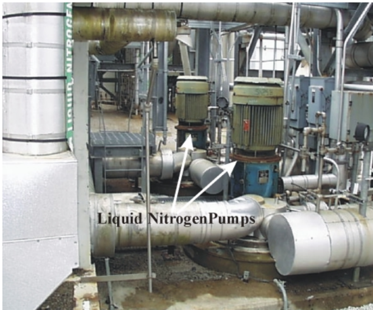
Figure 5.1.7A: Liquid Nitrogen Pumps
