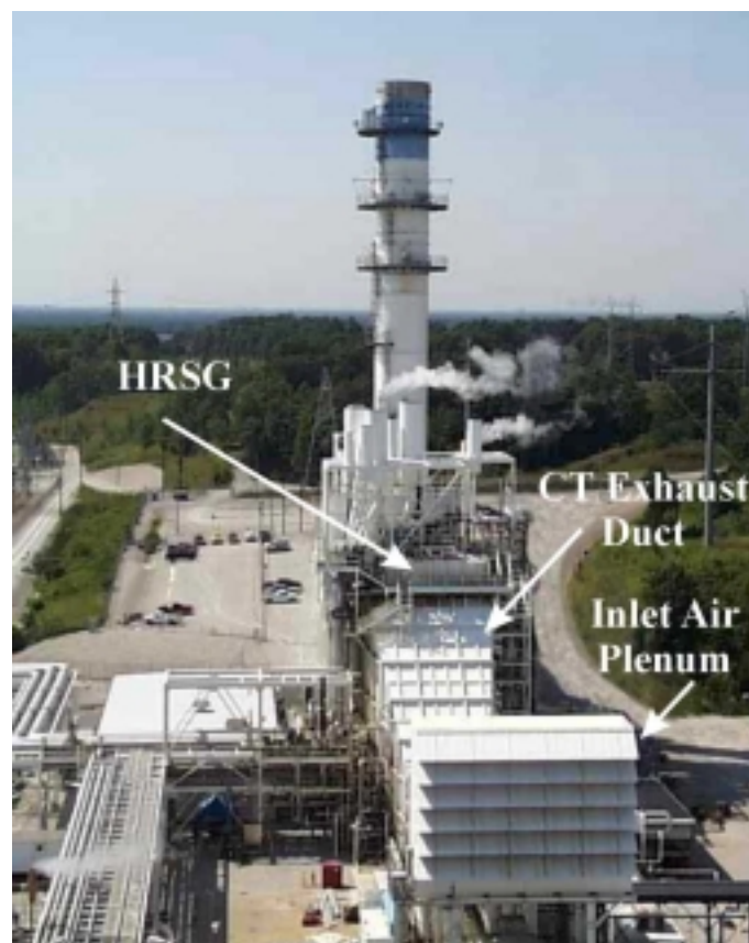
Figure 5.4.1A: Combustion Turbine
