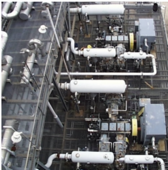
Figure 5.3.12C: Tail Gas Recycle Compressors
