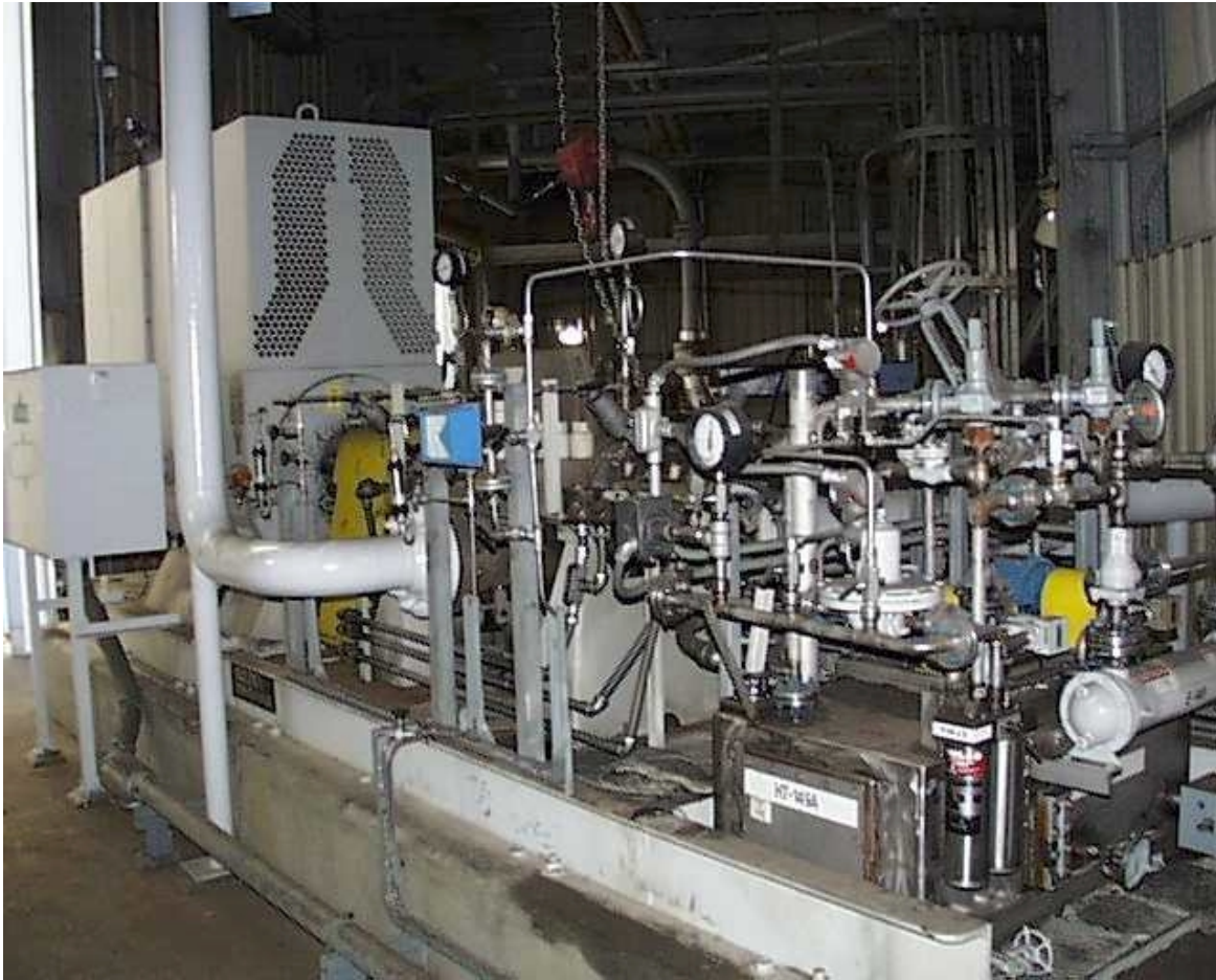
Figure 5.3.4D: Slag Quench Feedwater Pumps
