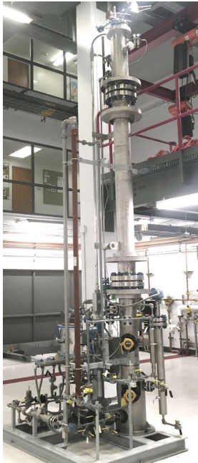
100 kW Prototype Staged Pressurized Oxy-combustor
