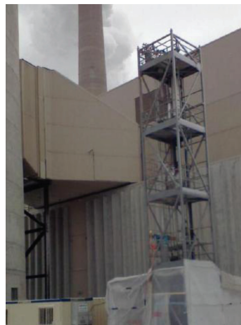
ADA-ES 1-kW Pilot-Scale Test Equipment
