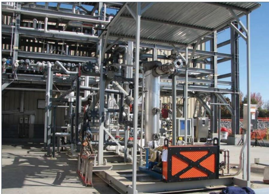
Figure 5: Membrane skid used for 1-TPD bench-scale slipstream testing at NCCC.
