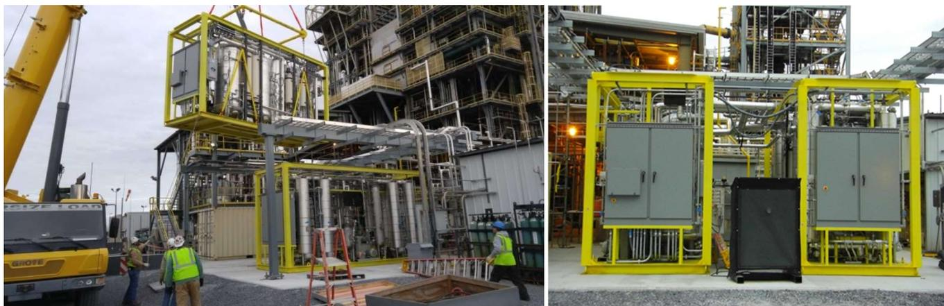
Figure 4: TDA's 0.1-MWe pilot unit installed in the test pad at the NCCC (Wilsonville, AL).
