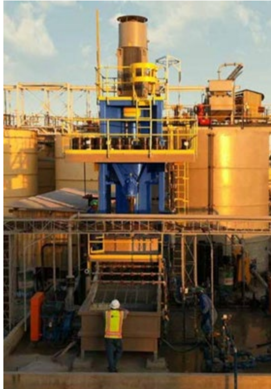
Figure 2-7 Typical VXPmill Installation
