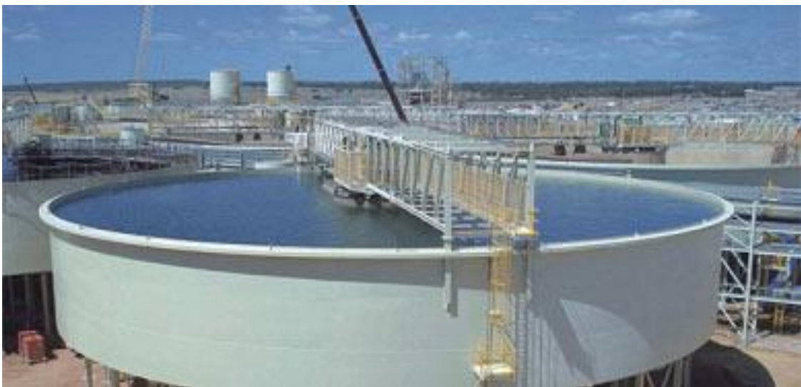
Figure 5-5 Typical Thickener Installation
