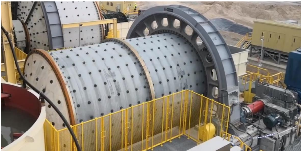
Figure 5-2 Typical Ball Mill Installation
