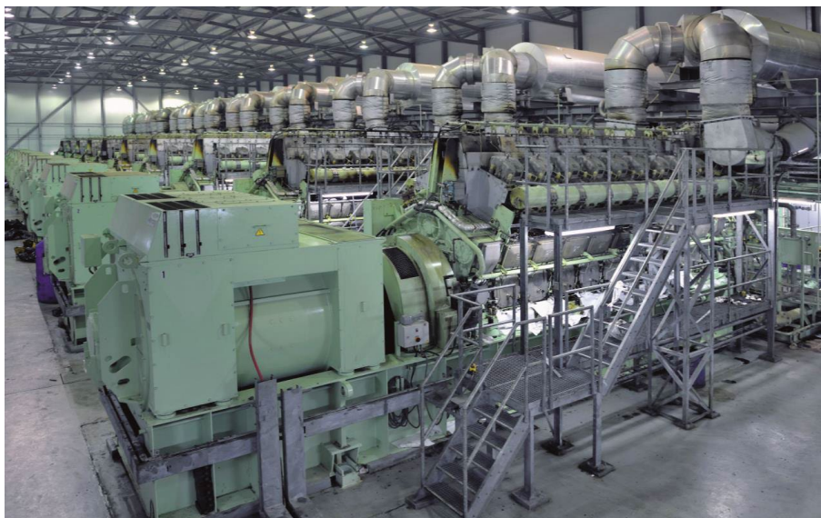
Figure 2 MAN gas engine generators (20 MW units at 500 rpm)
