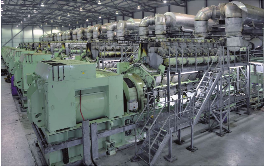
Figure 3-2 MAN Gas Engine Generators (20 MW, 500 rpm)
