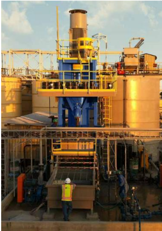
Figure 5-3 Typical VXPmill Installation
