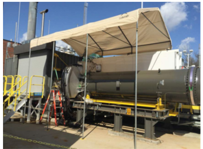
Figure 3. Photo courtesy LG Fuel Cell Systems
